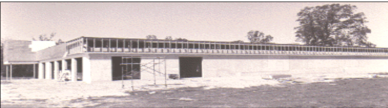
Construction of Data Services, Inc. in Winterplace Park.
