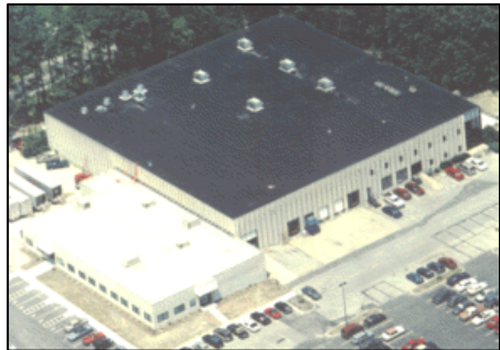
K&L Microwave recently purchased and renovated this 60,000 sq. ft. facility in Northwood, adjacent to the company's existing Northwood plant.
